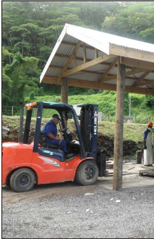
Forklift in action
